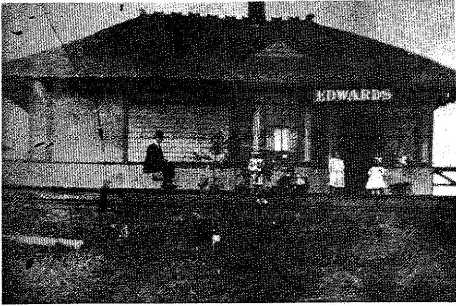
The Edwards Station
